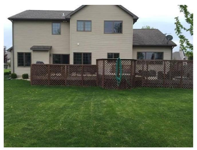
The original deck was dated, requiring extensive maintenance, and unusable. The team considered replacing the with low maintenance materials but the cost of composite decking lumber was not ideal. The deck had multiple levels that were too small to be usable. It had a privacy fence that blocked off the backyard, making both the deck and backyard seem small.
