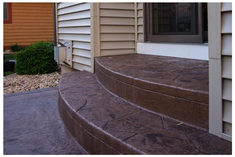
Two different patterns were used on the patio. Fieldstone was on the stairs to the patio door and firepit area; Chiseled Slate for the balance of the patio. A brick soldier course was used at the borders.
