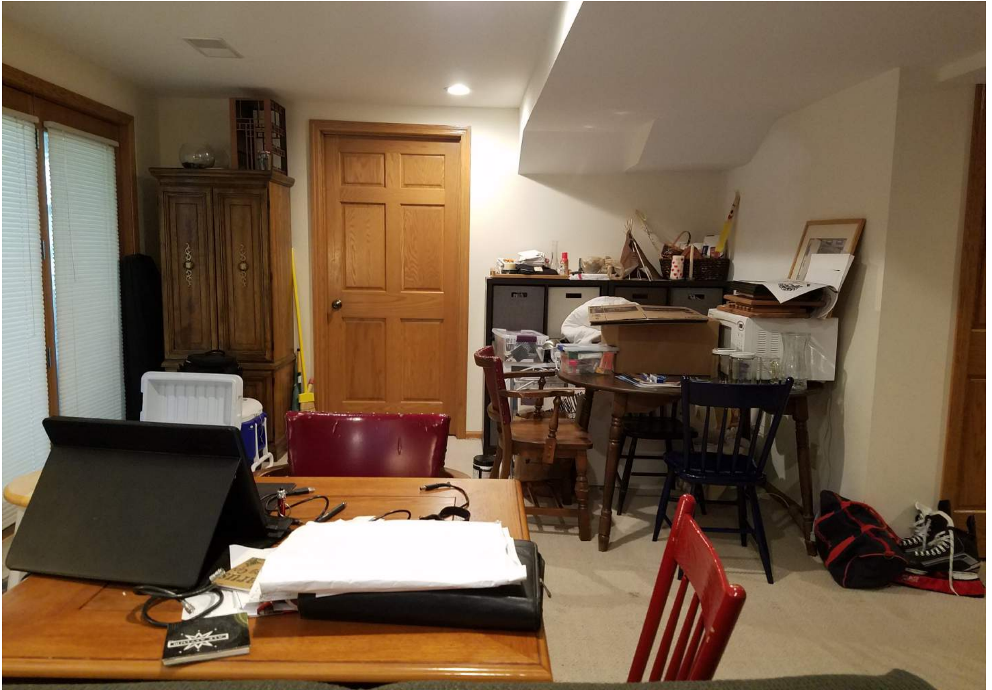
BEFORE: VIEW OF THE BASEMENT TOWARD THE MECHANICAL ROOM. CORNER USED FOR STORAGE.
