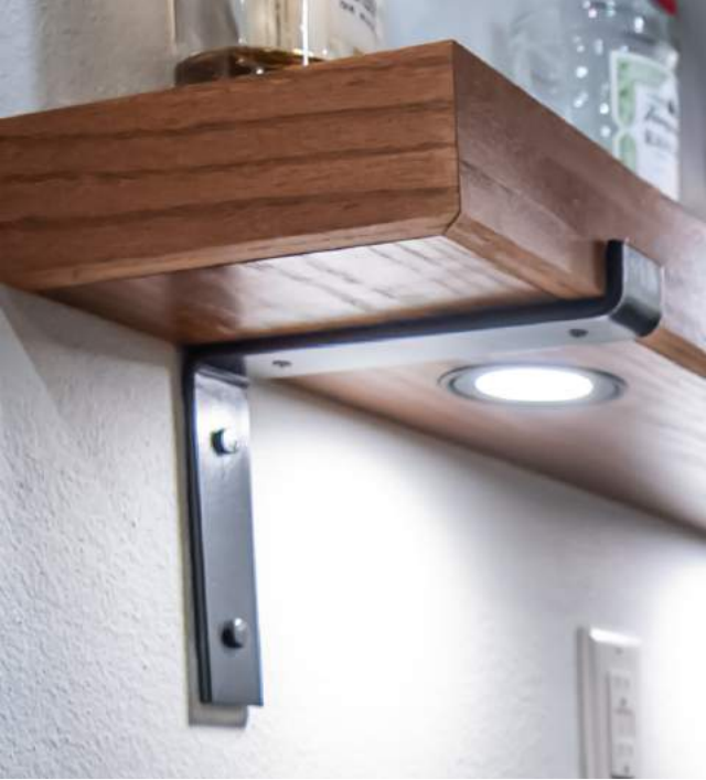
AFTER (ABOVE): DETAIL OF CUSTOM MADE FLOATING SHELVES WITH EXPOSED BRACKETS AND INTEGRATED LIGHTING.
