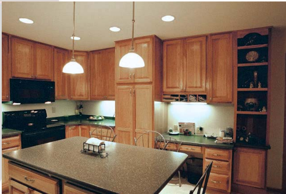
A combination of lighting options allows the space to be fine-tuned for work or for ambience. Fluorescent under-cabinet lights balance the energy usage of halogen recessed cans and incandescent pendants.
