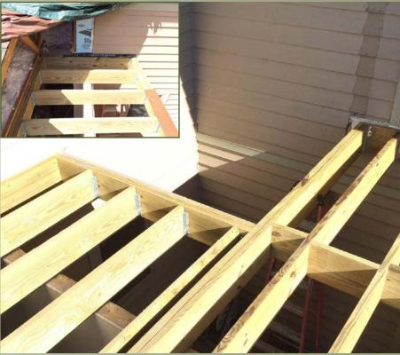
The footprint was expanded as far as possible without making structural modifications to the garage trusses.
